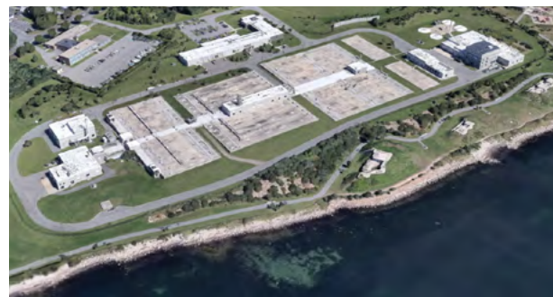
3. water treatment plant
