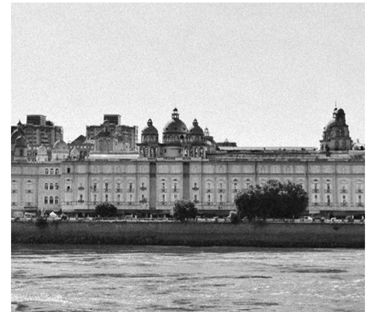
Figure 41. Central Island, Existing Condition
