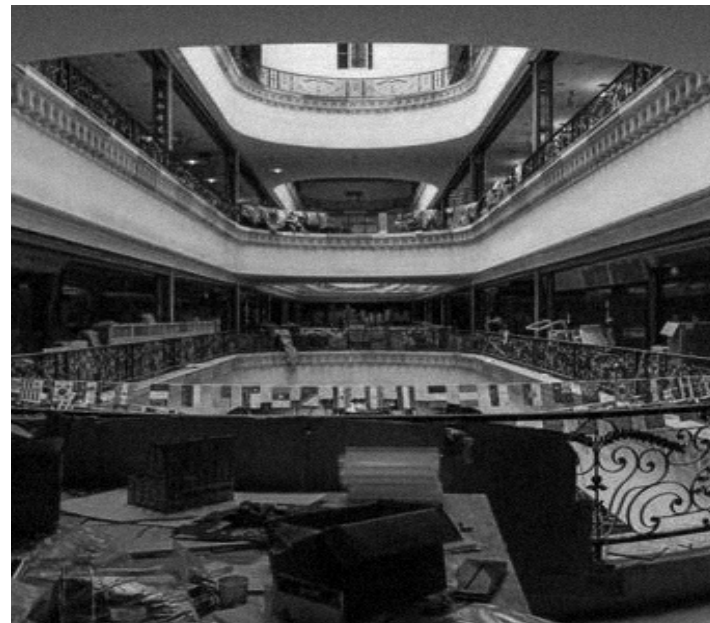
Figure 42. Central Island, Existing Condition
