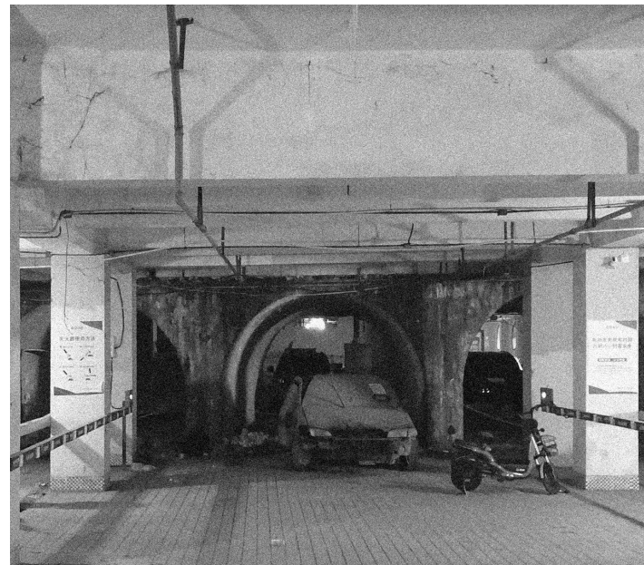
Central Island, Existing Condition
