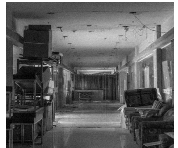
Figure 44. Central Island: Existing Condition
