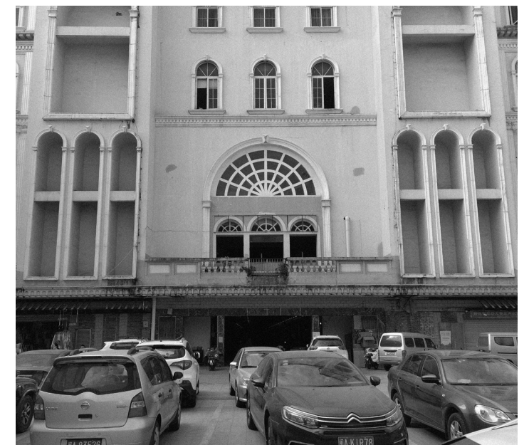
Central Island: Existing Condition
