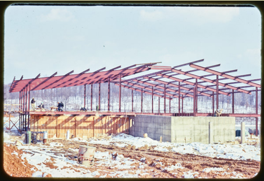
Photo of the Exhibition Center during construction, showing primary use of steel and concrete. Major feature of tilted red roofs with space in between.
