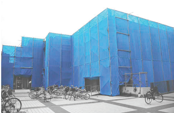
Construction Site II - Tsukuba-shi
