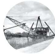
Dredging Miami Canal
