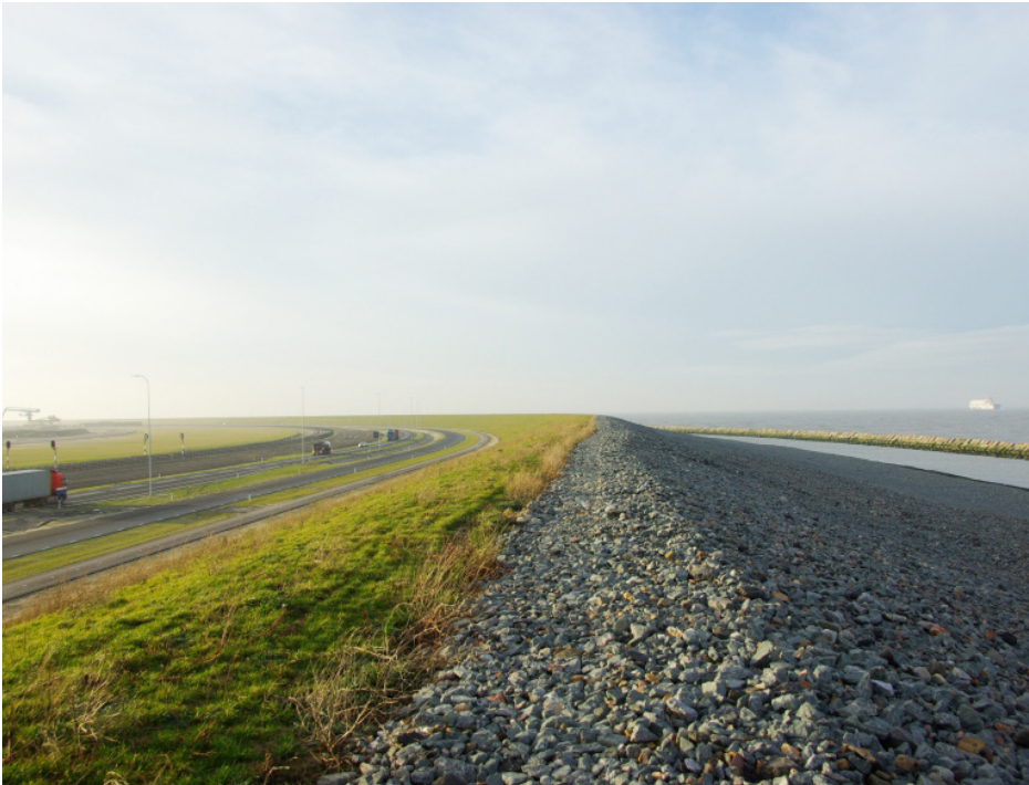
Storm protection barrier around port of Rotterdam, Rotterdam 14
