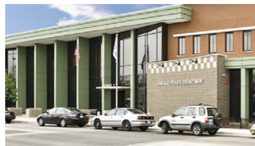
Dicing is often used as signage, and architectural detail on newer police stations.
