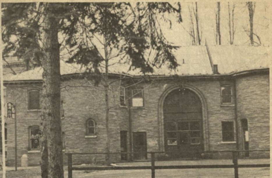
1895 Carriage House, Cabana Estate, 824 Delaware Ave, now used as a school for Children's Aid. Threatened to be replaced by the parking lot.
